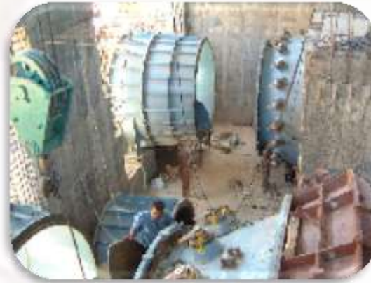
PLANT Installation FOLLOW UP
