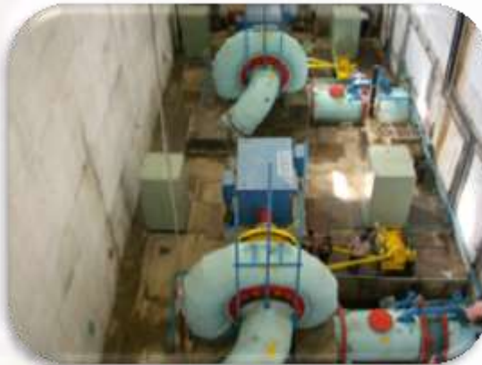
PLANT Installation FOLLOW UP
