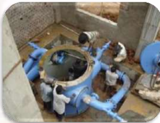
PLANT Installation FOLLOW UP
