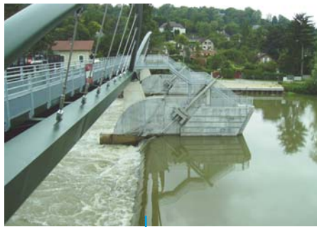
Dam of L'Isle Adam (France) 7 Hydraulic Cylinders DA 280 x 130, Stroke 5 600 mm
