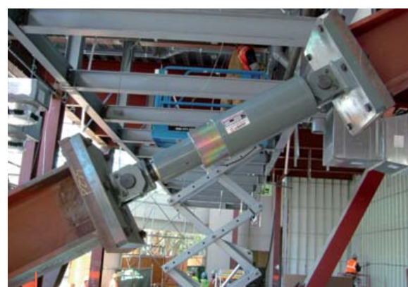
Viscous fluid dampers ASR 1500-108 AH 200 Kips, 4.0 in. +/- Stroke, a = 0.1
