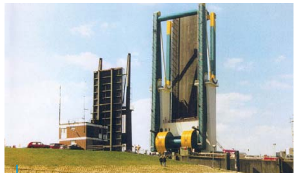
Estesperrwerk Mobile Bridge (Germany) Rods in KERADOUCE® coating 2 Hydraulic Cylinders DA 500 x 360, Stroke 10 600 mm 4 Hydraulic Cylinders DA 460 x 280, Stroke 7 700 mm 2 Hydraulic Cylinders 63 x 36, Stroke 320 mm 4 Hydraulic Cylinders 100 x 70, Stroke 500 mm 4 Hydraulic Cylinders 100 x 70, Stroke 1 600 mm
