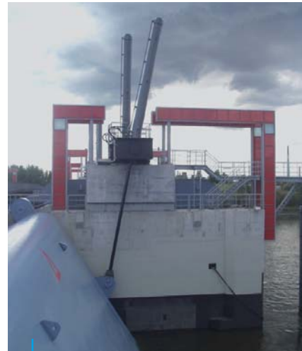
Billwerder Bucht Dam (Germany) - Rods in KERADOUCE® coating 16 DA Hydraulic Cylinders 560 x 220, Stroke 8 400 mm
