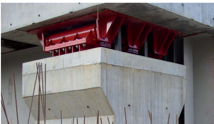
Longitudinal preloaded spring dampers on abutment High speed railroad bridge of Epenottes, France RAP longitudinaux sur la culée - Viaduc des Epenottes TGV Rhin-Rhône
