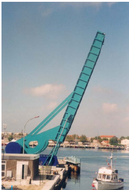
Mobile Bridge + Sluice Gate 2 Hydraulic Cylinders 250 x 200, Stroke 5 760 mm
