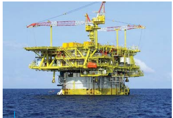
Murphy Kikeh : 73 Production Riser Tensioners Dia. 260 x 110, Stroke 6 403 mm with 1 low pressure accumulator (20 gal.) + 2 high pressure accumulators (110 gal. each)
