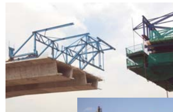
Chalifert High Speed Train Viaduct (France) Douce-Hydro's lifting and launching systems push the bridge deck. A total of 32 000 tons of deck was pushed over 3,2 km, allowing the construction of the high speed train rail tracks. 4 SA Hydraulic Cylinders dia. 530 mm, Stroke 70 mm 8 DA Hydraulic Cylinders 250 x 180, Stroke 250 mm 8 DA Hydraulic Cylinders 110 x 75, Stroke 1 000 mm 8 power packs + 4 sets of general mechanism
