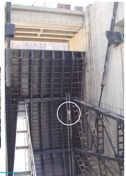
10 Hydraulic Cylinders for radial gates DA 400 x 160, Stroke 17 500 mm with rods in KERADOUCE® coating
