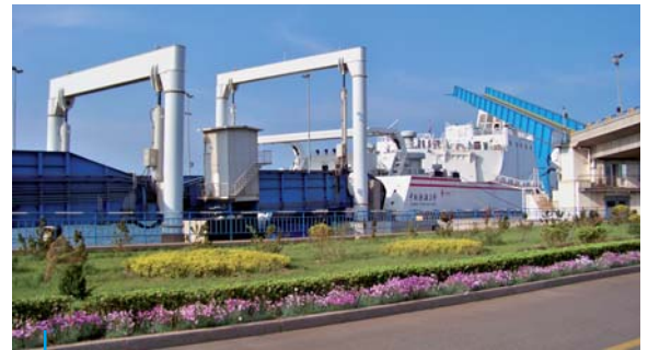
Seaport linkspan Cylinders
