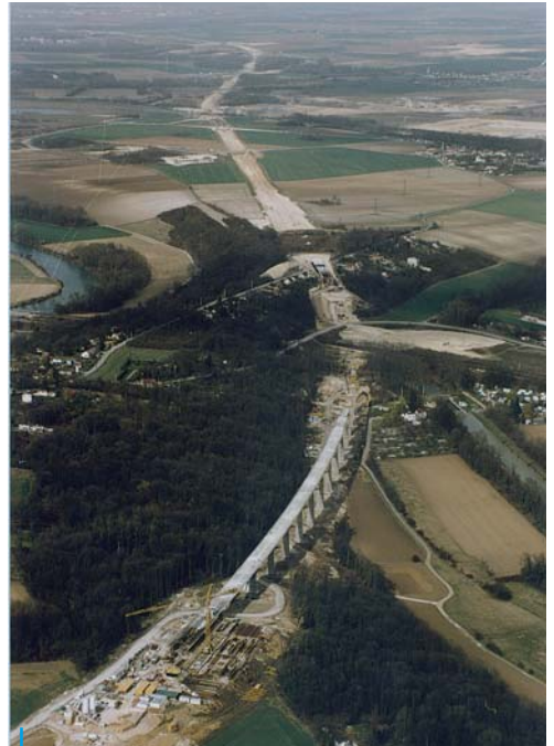
Chalifert High Speed Train Viaduct (France) Douce-Hydro's lifting and launching systems push the bridge deck. A total of 32 000 tons of deck was pushed over 3,2 km, allowing the construction of the high speed train rail tracks. 4 SA Hydraulic Cylinders dia. 530 mm, Stroke 70 mm 8 DA Hydraulic Cylinders 250 x 180, Stroke 250 mm 8 DA Hydraulic Cylinders 110 x 75, Stroke 1 000 mm 8 power packs + 4 sets of general mechanism
